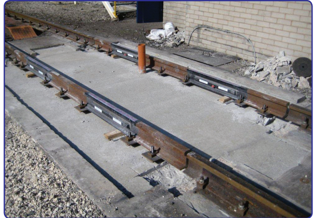
Weighline transducer rails being installed
