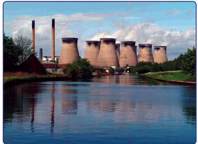
View of Ferrybridge Power Station
